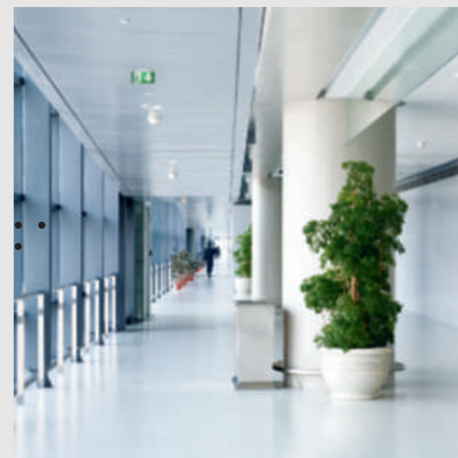
X-Light 360 ensures evacuation lighting with perfect integration.
