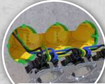
Installation of pre-wired sockets
